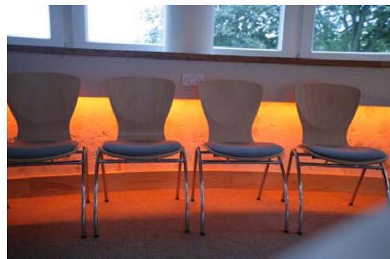
The half wall above conceals cables as well as provides the perfect mounting location for linear amber LEDs that are run on Direct Current – a gentle effect akin to candlelight
